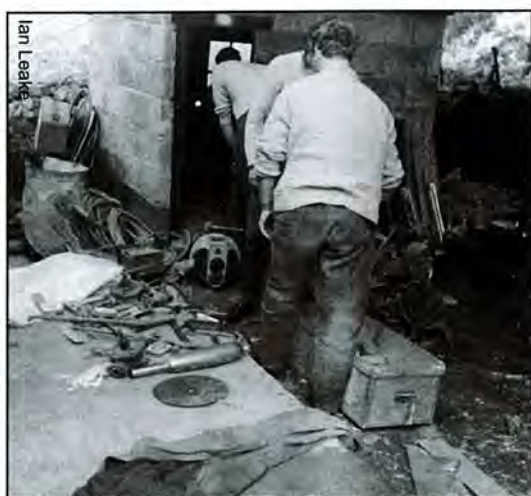
Installing the generator in the genny-shed
